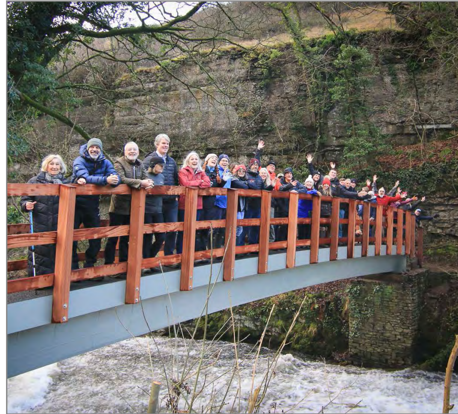
Picture credit: R&C Williams, Cressbrook Footbridge
