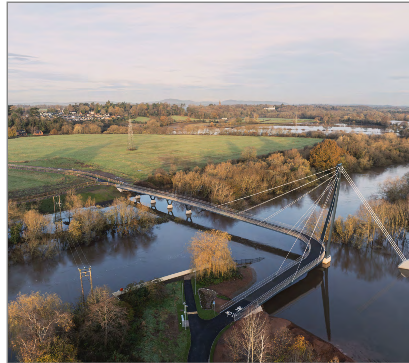
Picture credit: Kepax Footbridge, courtesy of Alun Griffiths
